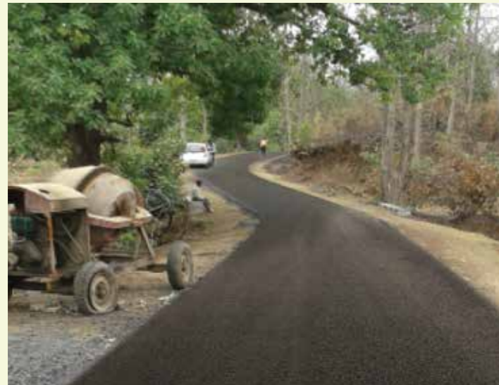
Figure 3. After Cold mix Application
