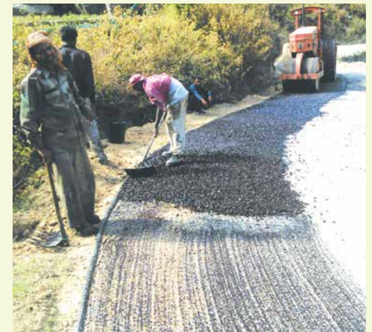
Figure 2. Cold Mix being laid
